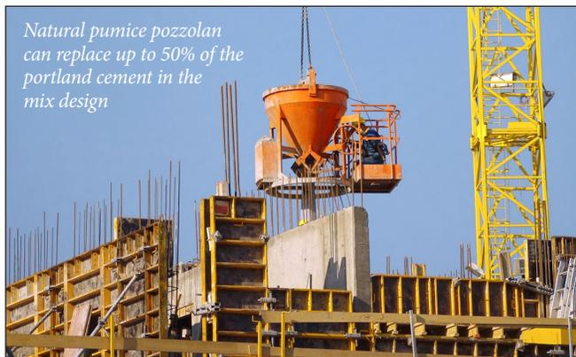
Natural pumice pozzolan can replace up to 50% of the portland cement in the mix design
